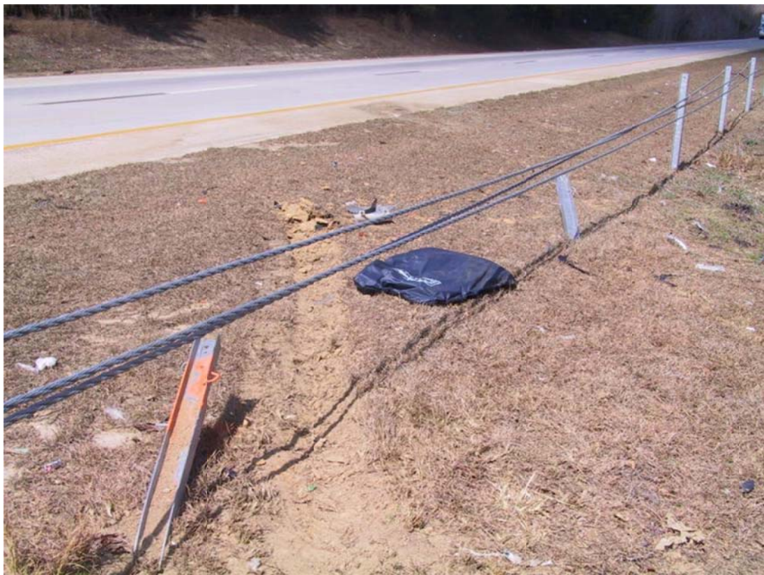
Figure 94. Diving Underride Penetration Crash in North Carolina
