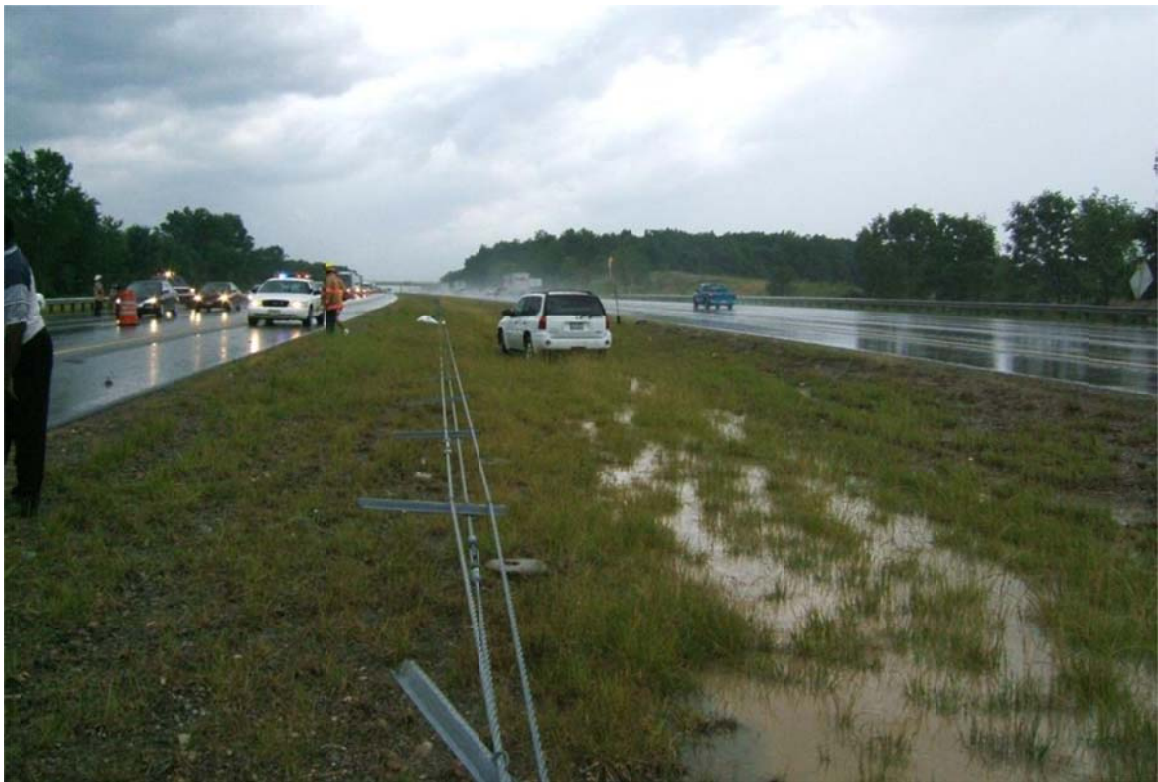
Figure 83. Override Penetration Crash Caused by Strong Cable-to-Post Attachment
