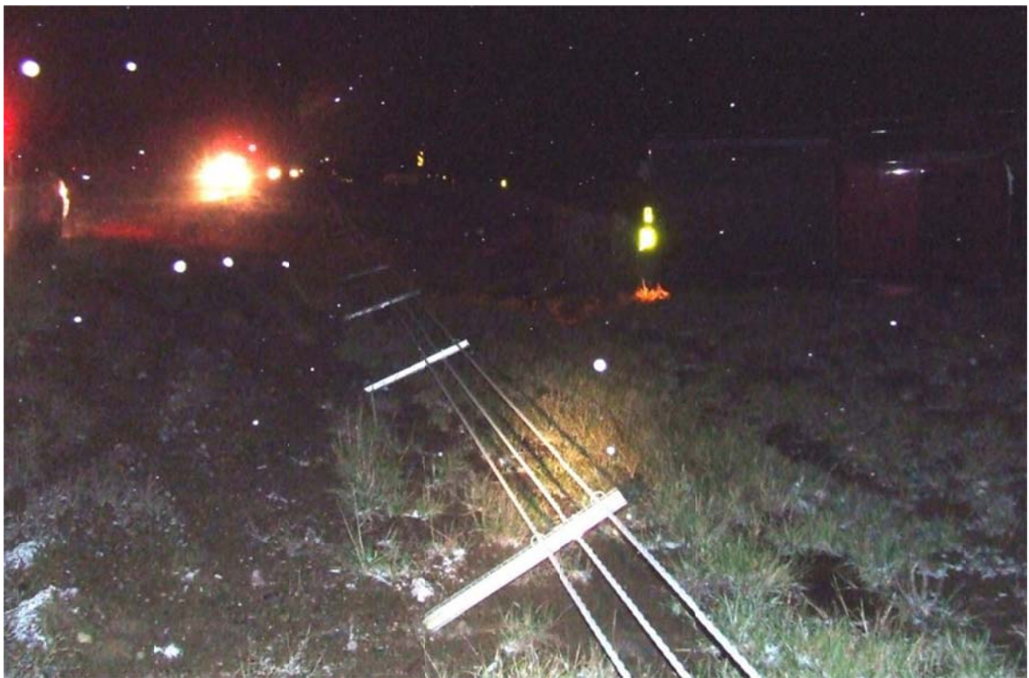
Figure 81. Penetration Crash Caused by Strong Cable-to-Post Attachment
